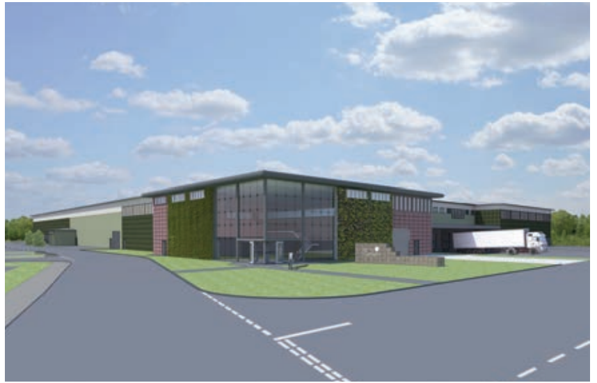
An artist's impression of the new Berry Gardens packhouse at Linton near Maidstone, Kent.
